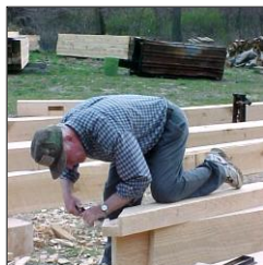
Jack Romesberg work on a brace
